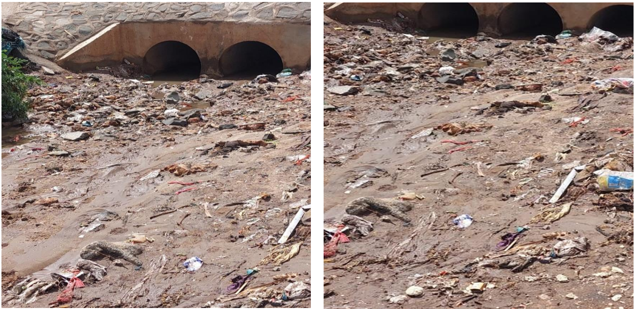
Figure 5: Clogged Storm Water Drainage systems in Kajiado town
