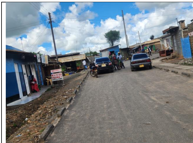
Tarmac Road and Row Housing in Majengo
